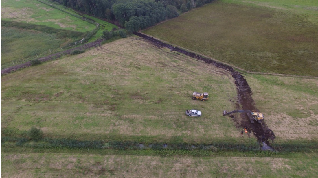
Construction of watertight membrane on north-western border of Purker Fenner.
