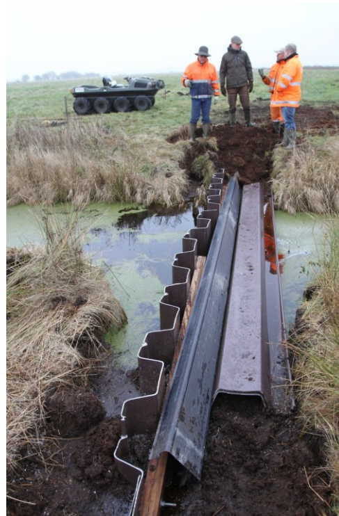
New weir replacing the pump
