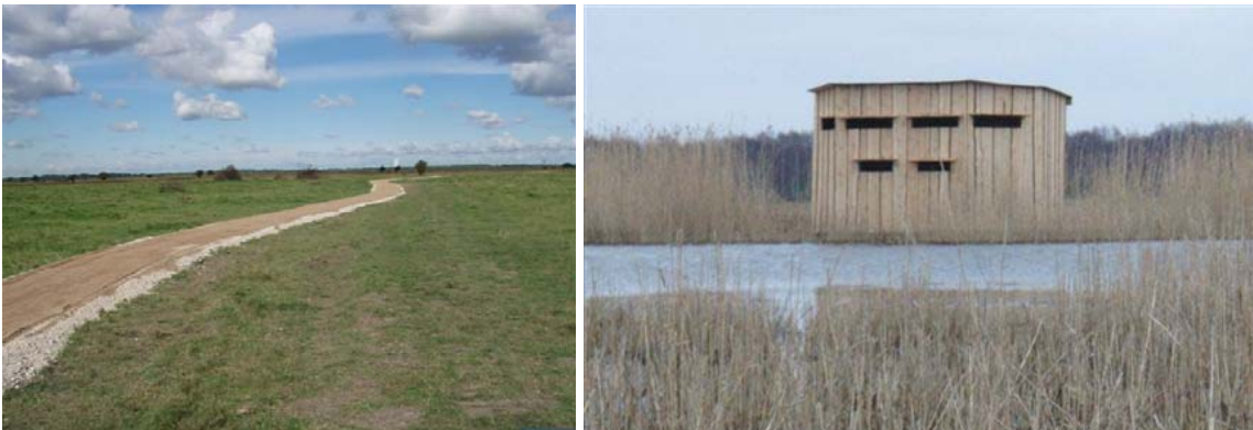
The foot path and the bird observation platform at Vestamager
