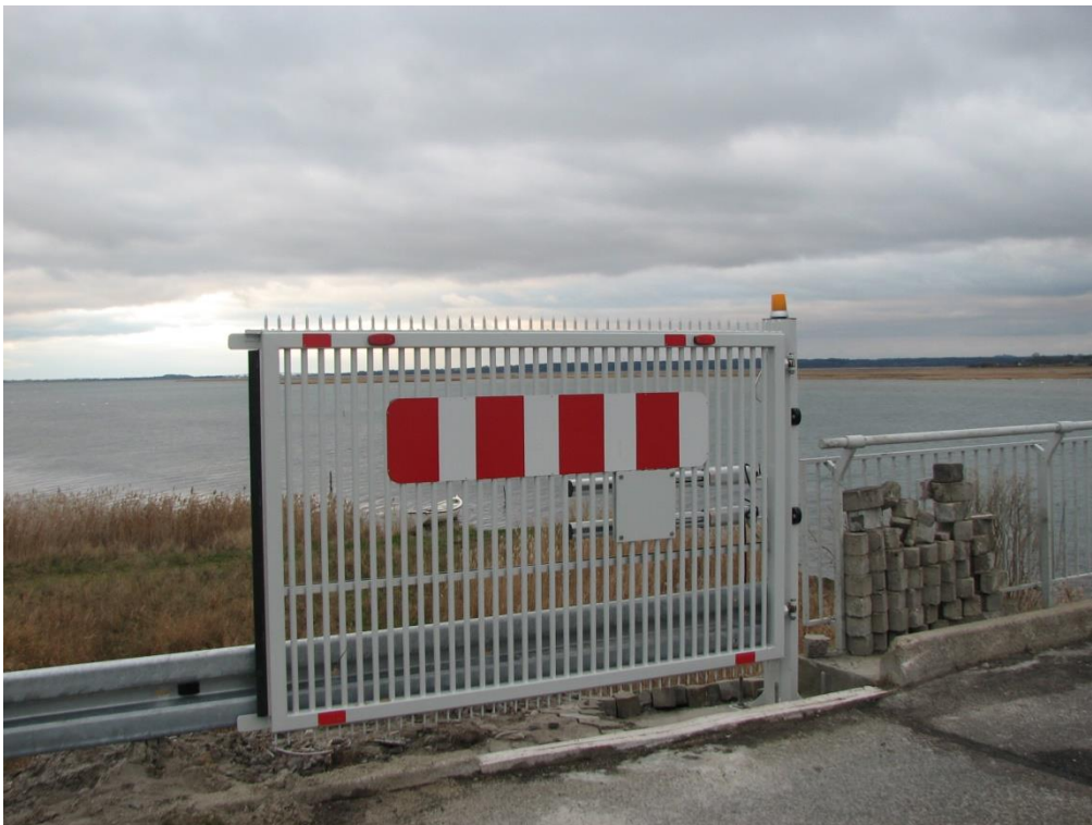
Picture 6: The gate on the bridge between Møn and Nyord. The gate is 1.5 m high and made of a steel frame of only vertical bars with a maximum free distance of 40 mm. It is raised 15 cm above ground in order not to push snow into a heap when opening, and under the gate frame there are vertical spikes, which cut through the snow but prevent foxes from creeping under. Picture by Jørgen Sandby Nielsen.
